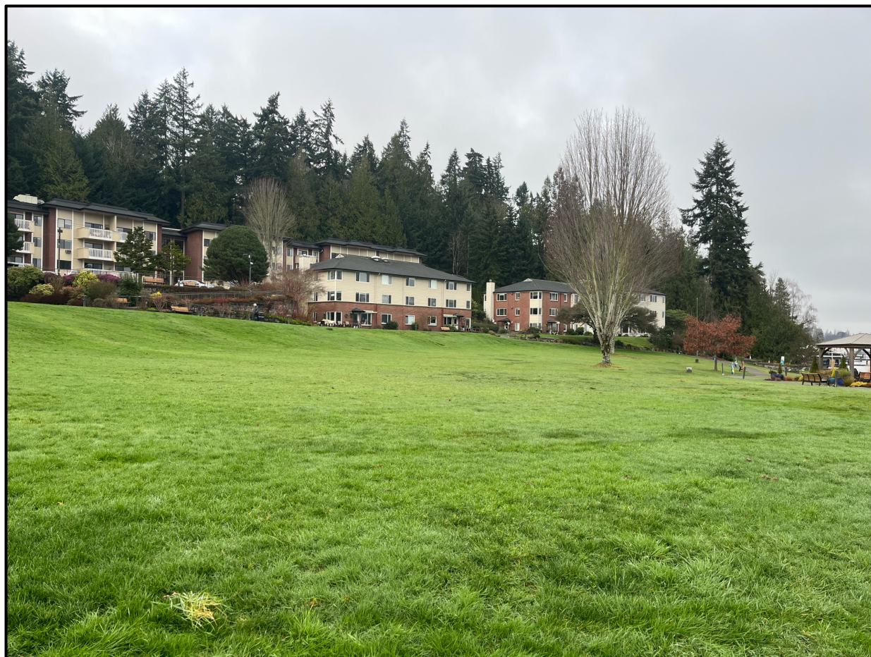
Figure 5 - Looking Northwest Towards On-Site Residential Structures
